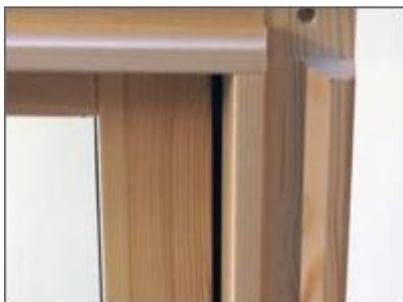
To make sure the frame is set properly, check the gaps at the closure of the sash. If the vertical gaps are parallel with the gap at the bottom in a slightly opened position, then the frame is correctly aligned, and the top brackets can be fixed.
